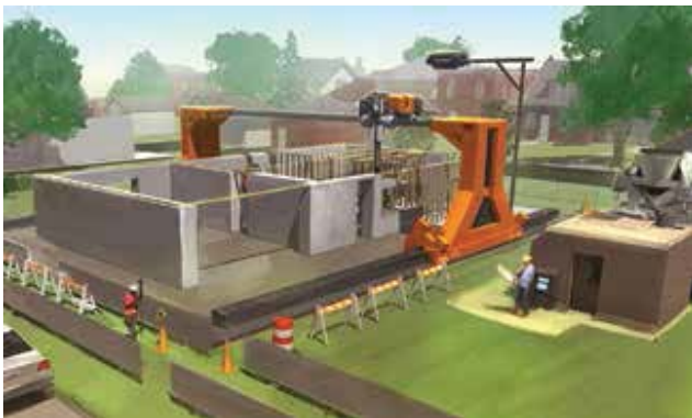
Figures 1 and 2. Contour Crafting “24 Hour House” and a panel prototype being fabricated. Images: Dr. Berok Khoshnevis, professor, University of Southern California.
